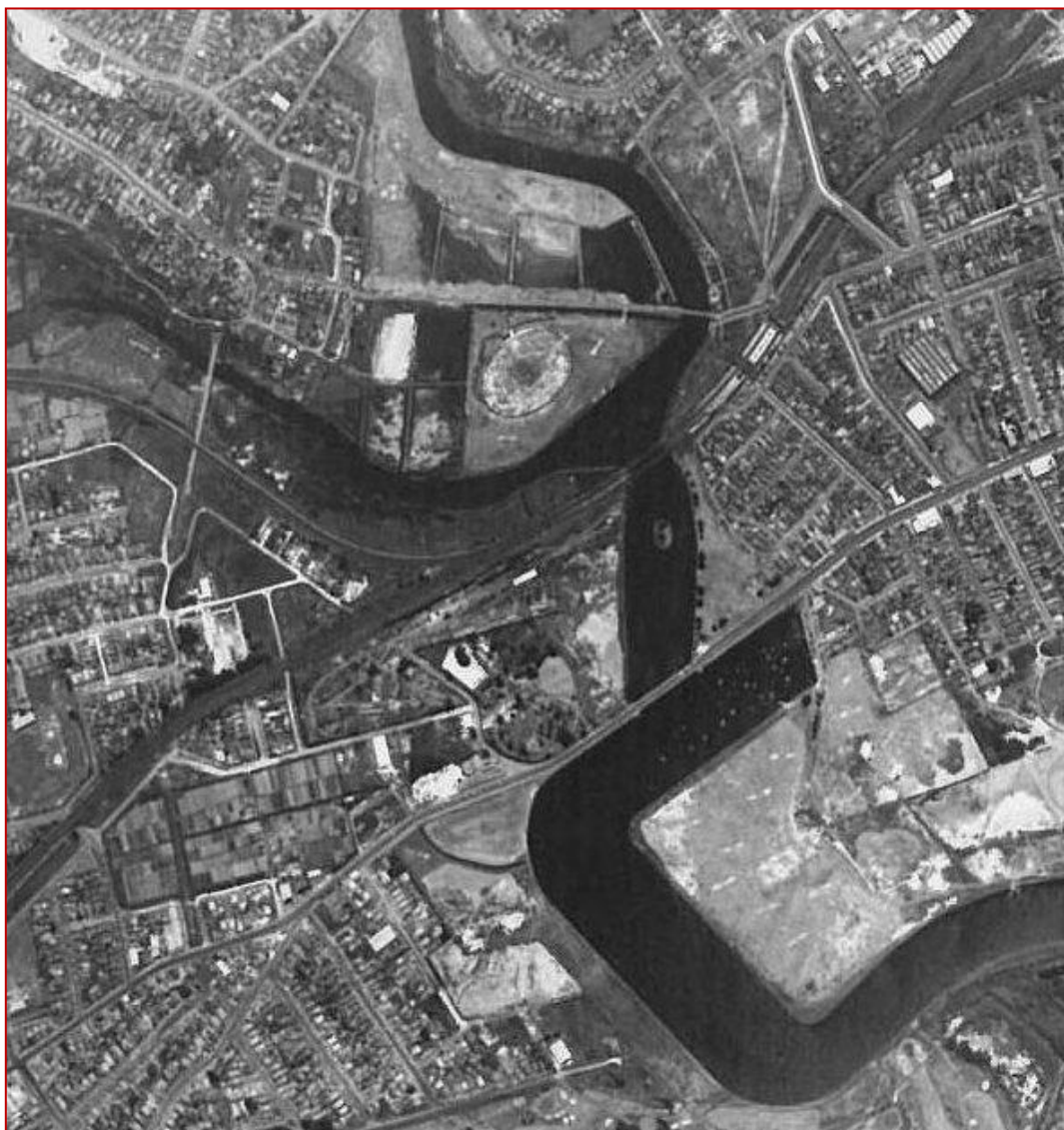
Figure 62 Aerial photograph of works associated with Sydney Airport, 9 February 1951. The weir WC17 is not present (Source: Madeline and Warren Ide Collection through Aadastra Aerial Surveys)
