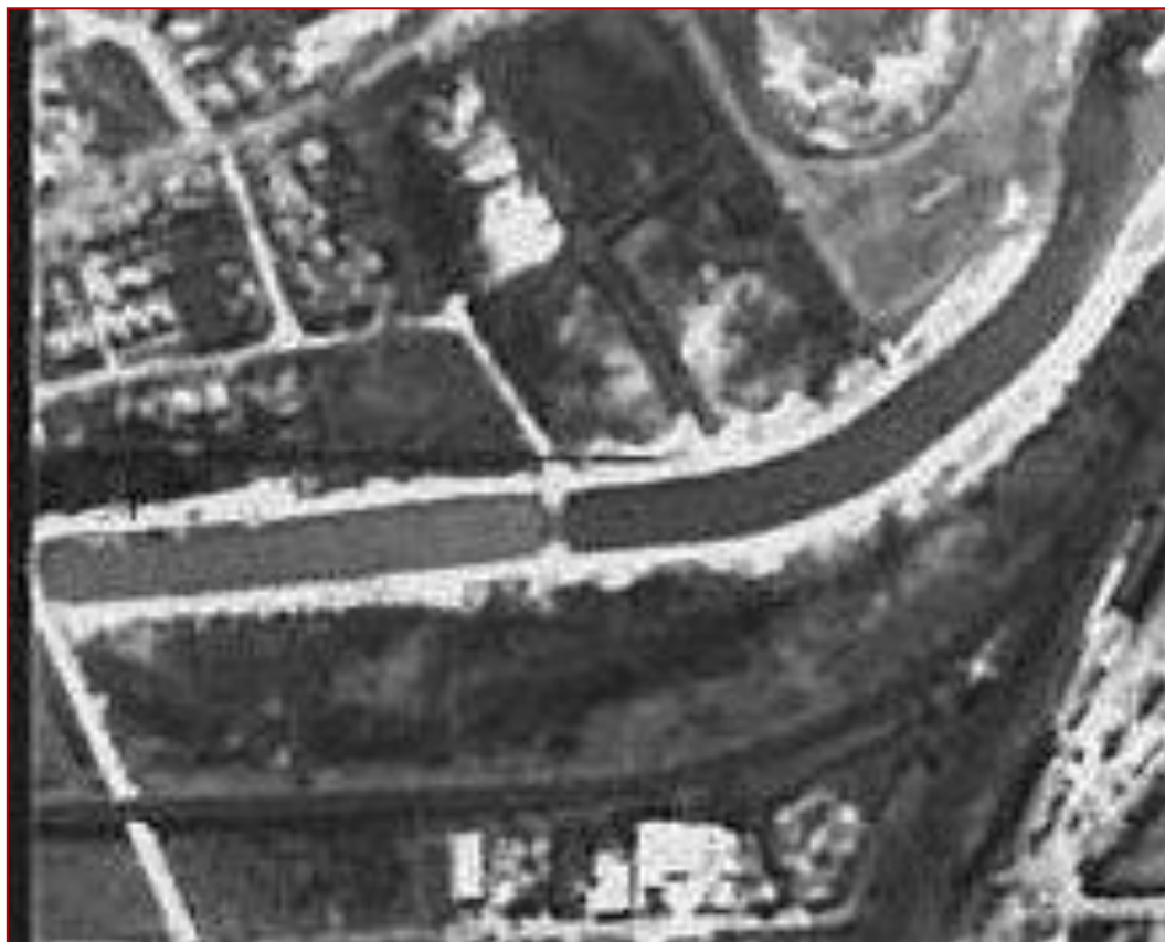
Figure 64 Detail of 1952 image showing the weir (centre)
