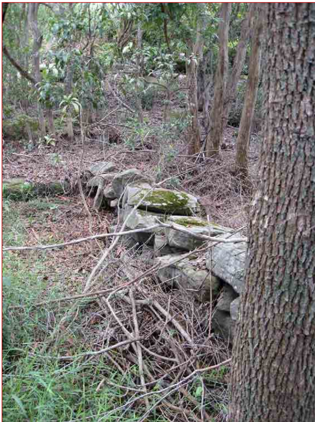
Figure 45 2015 WC10 looking west
