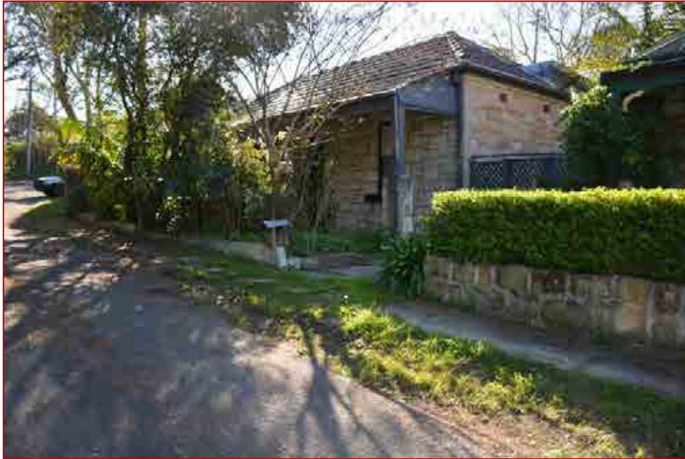
Figure 42 One of the Jackson Place cottages, looking northwest
