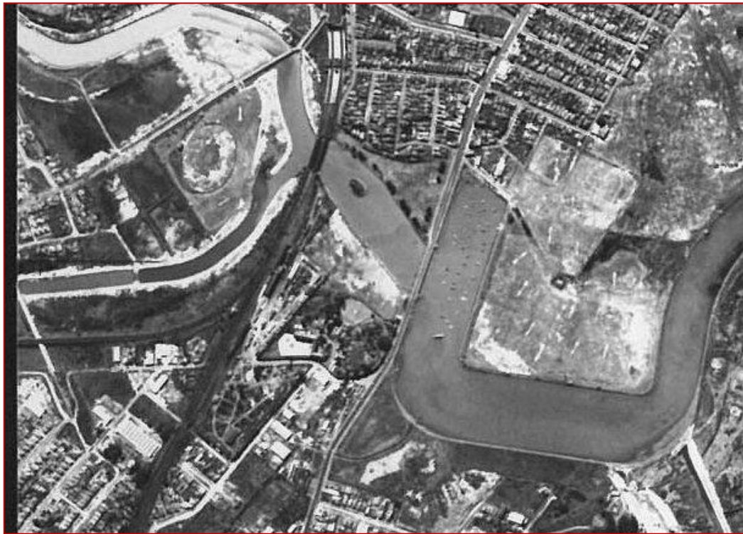
Figure 63 Aerial photograph of works associated with Sydney Airport, 18 April 1952. The weir WC17 is clearly visible to the right of the aqueduct (Source: Madeline and Warren Ide Collection through Adastra Aerial Surveys)
