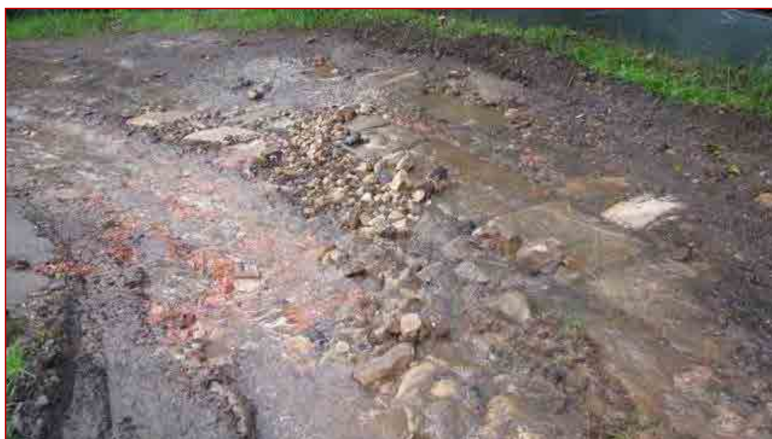
Figure 20 2014 WC2 Brick rubble and flagging (WCPS)
