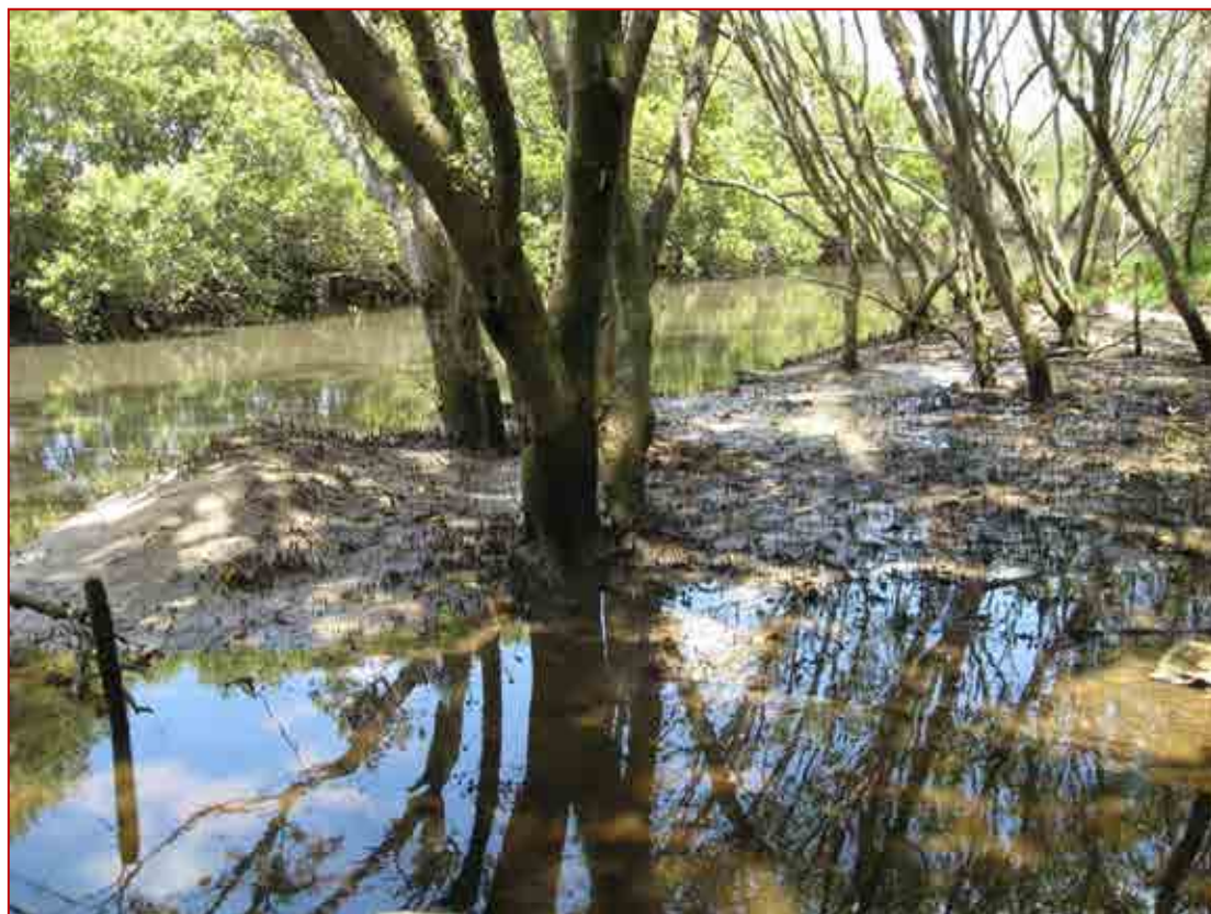
Figure 50 WC11, eroded southern bund, 2015
