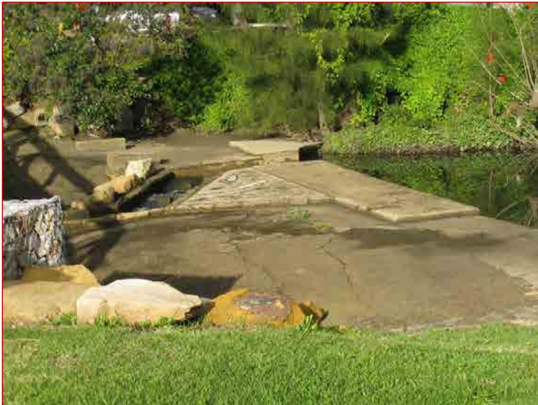
Figure 40 WC7 weir looking south
