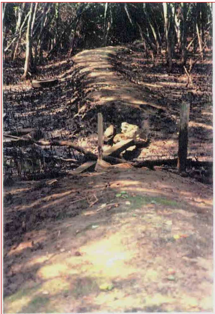
Figure 47 WC11, eastern bund looking south, 1992
