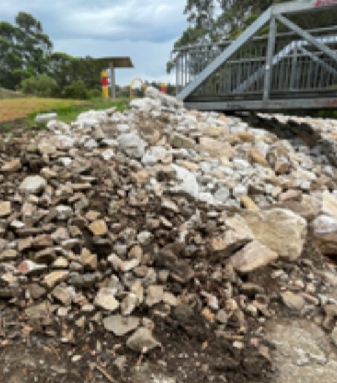
Boulders and original gabions at footbridge
